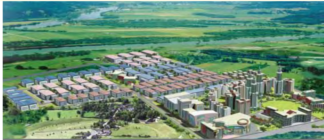
Kanchan Janga Integrated Park, Siliguri | Total built-up area: 3 million sq.ft.
